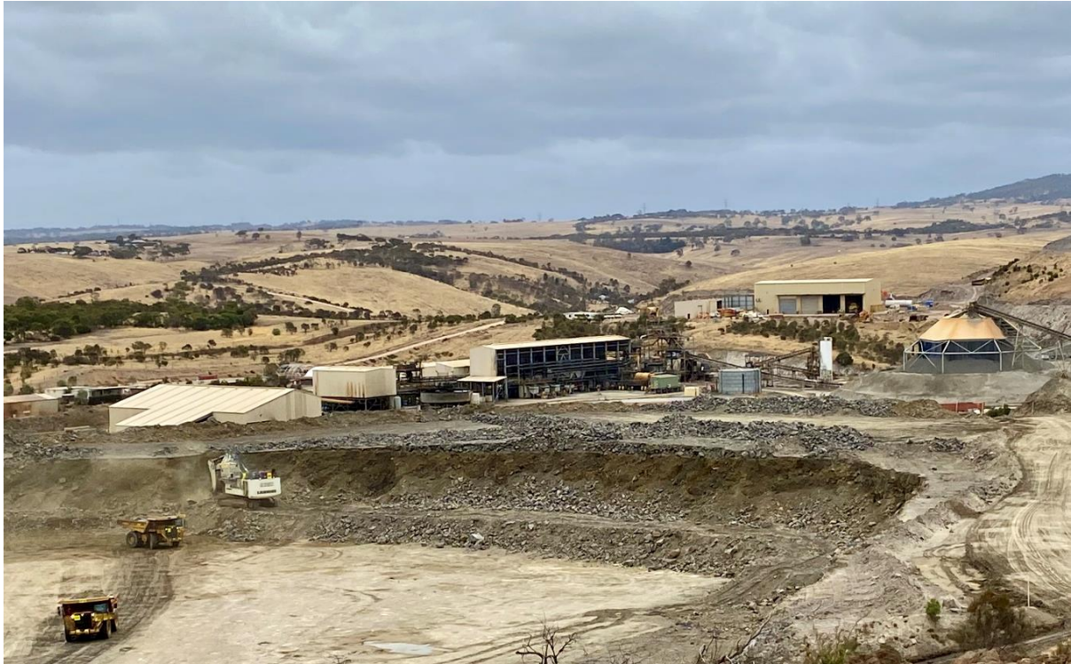
FIGURE 2. RECLAIMING ORE STOCKPILE
