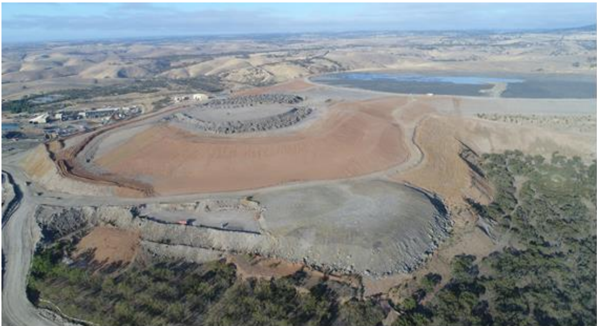
FIGURE 3. TOPSOIL SPREADING ON SHAPED LANDFORMS IN PREPARATION FOR SEEDING
